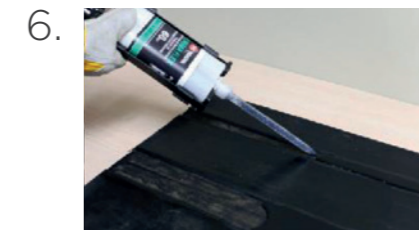
6. Apply Permaflex repair material
